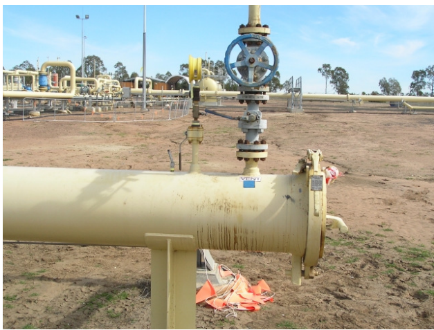
Pig receiver and sampling point
